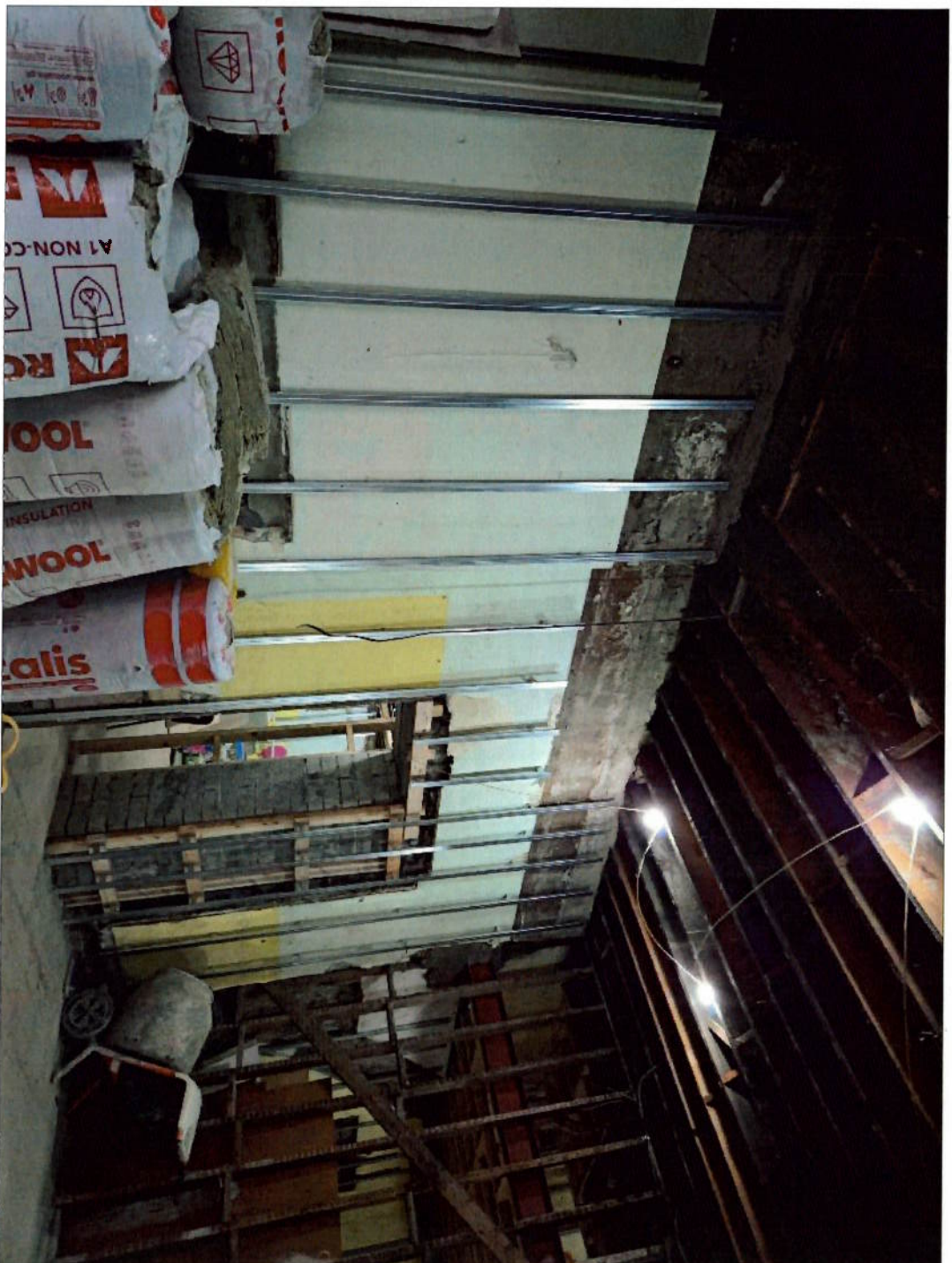
View 8: Typical Internal Works
